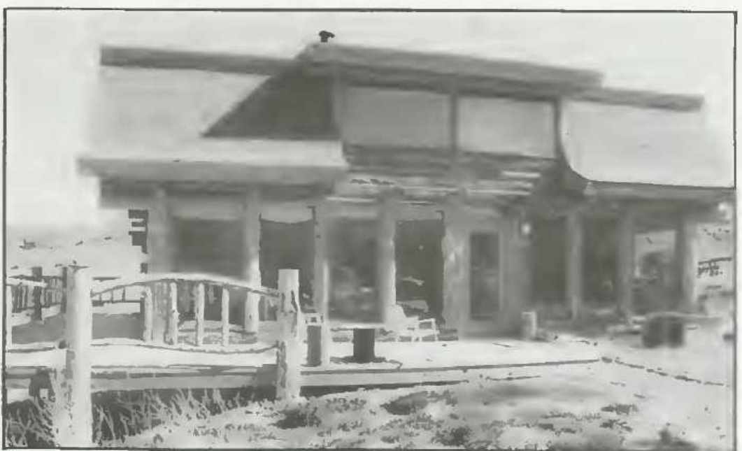
At 5,700 feet elevation, cold winters are the norm for Virginia City, but that doesn't bother Stephanie Wood. She gets most of her space heat from the almost-daily sunshine coming through her large south-facing windows.
