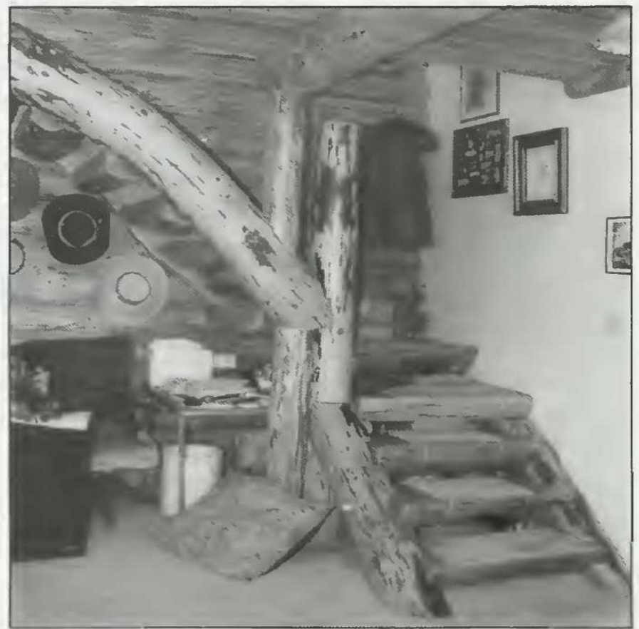
The house reflects the owner's liking for curved structures. A curving log staircase leads to the spacious bedroom and bath occupying the second floor. Crooked Douglas fir log uprights support the main beams. Outside, curved railings surround the deck wrapping the south and west sides of the house.
